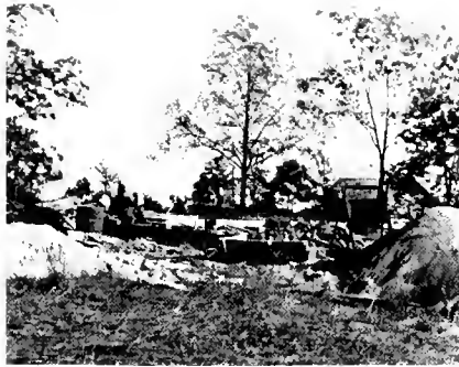
New Water Line
